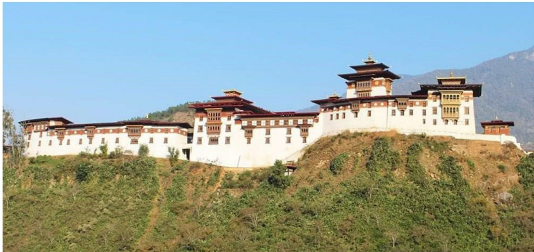
Wangdue Phodrang Dzong being restored to its glory
